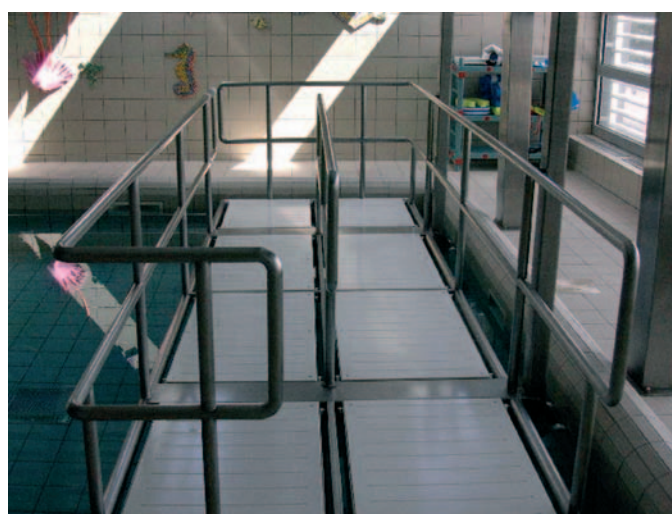
Figure 10. Couloir de marche double.
